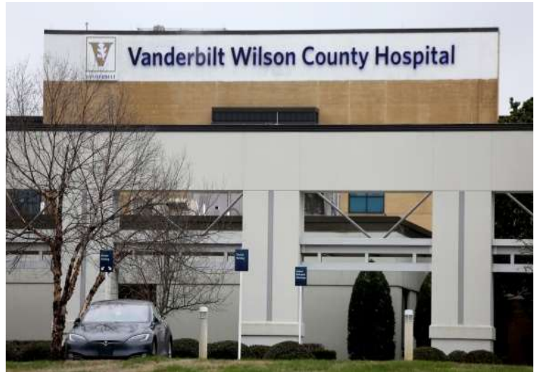
Vanderbilt Wilson County Hospital Main Hospital 1411 W Baddour Pkwy – Lebanon, TN
